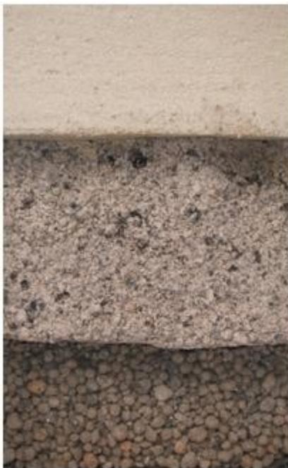
The Screed is normally 25 - 50mm thick; if you are laying underfloor heating then the screed will need to be 75mm thick.
