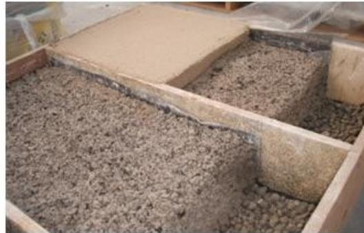
The curing times and requirements of the screed are as per the slab. In addition if you have installed underfloor heating you cannot use it for a minimum of 4 weeks.
