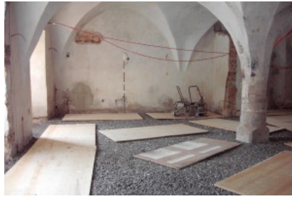
Glasscrete Floor Sub-base
