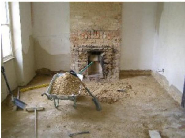
1. The first job was to dig down to the required depth for the Loosefill insulation and the limecrete slab.
