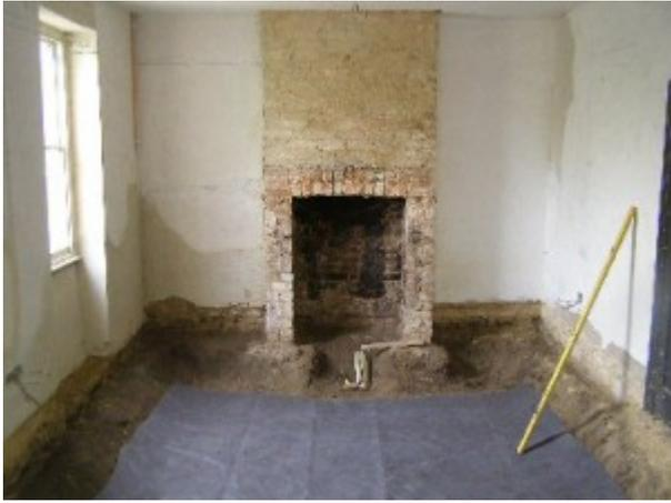
3. After removing 10 tonnes of soil by hand the next job was to lay the geotextile membrane to contain the loosefill
