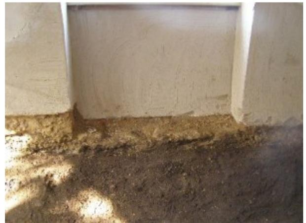
2. When digging down it was done at a slight angle so as not to disturb the foundations (or lack of!)
