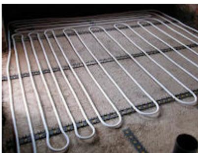
You can install underfloor heating when using limecrete, normally the pipes are tied to a geogrid mesh or fixed via a clip rail to the slab. Do not use a plastic sheet system that you clip the pipes into that can seal the floor like a DPM does.
