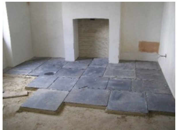
8. The flagstones being laid as a finish
