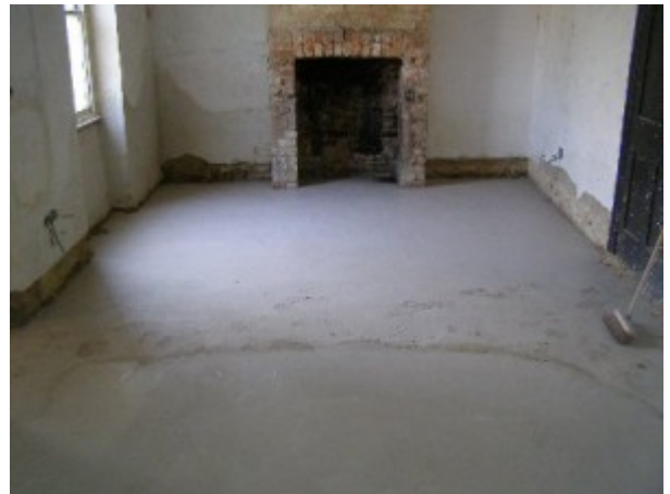
6. The finished screed
