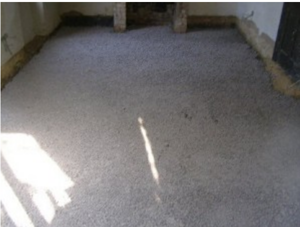
5. The completed Limecrete slab
