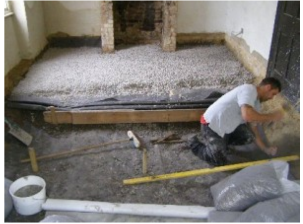
4. The loosefill & limecrete was laid in stages
